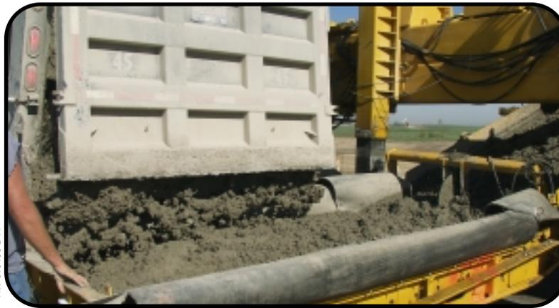
The GOMACO-designed conveyor system on the PS-4000 provides quick, clean and efficient delivery of concrete to the grade. The 5 ft. (1.52 m) wide GOMACO twin conveyor systems are built with the strength and durability to catch the concrete load from end-dump trucks.
